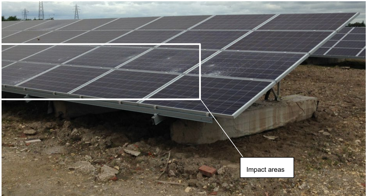
Plate 11.4: Vandalised PV Arrays, Thorne Solar Farm, Doncaster (as-built survey, L. Nevins 2016)
